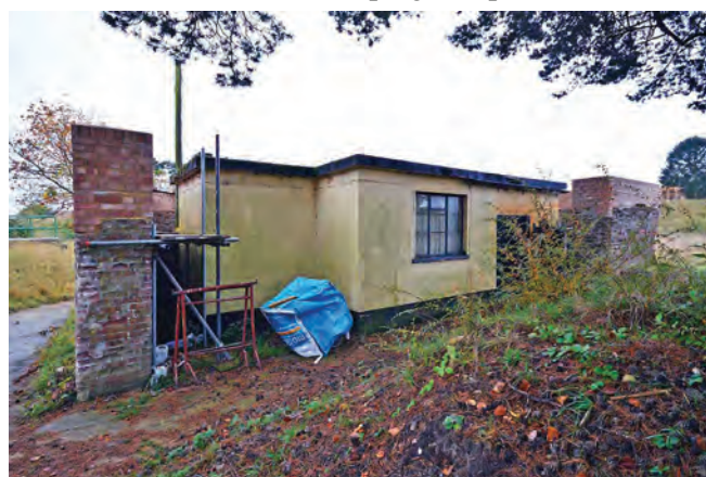
Core Inspection Building with its 0.7m thick surrounding blast wall
